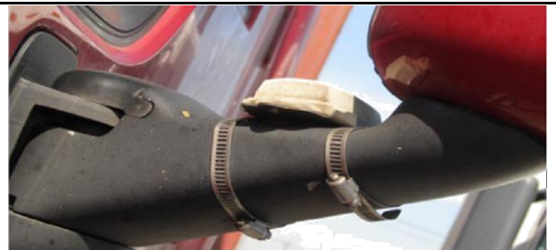
Large Clamp Installation
